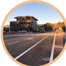
MARSH ST BRIDGE COMPLETED JANUARY 2021
