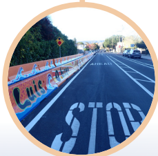
2020 ROADWAY SEALING (IMPROVEMENTS TO 82 ROADS SPANNING 19 MILES) COMPLETED OCTOBER 2020
