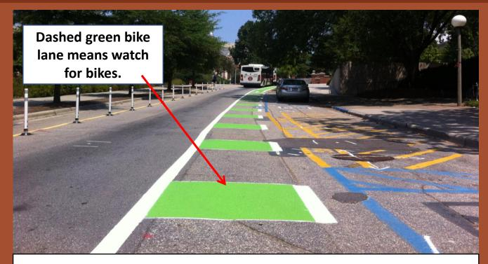
Transit stops will function the same was they do now, with buses pulling all the way up to the curb. Watch for bikes when pulling into and out of bus stops. These bike/bus mixing zones will be marked with dashed green bike lanes.
