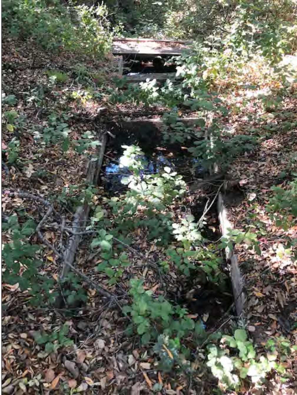
Figure 4-7 AE-4087-01H, concrete settling pond, facing south.
