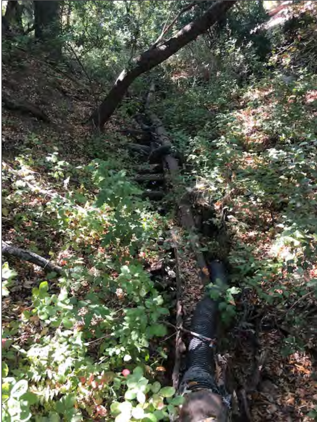
Figure 4-8 AE-4087-01H, steel pipeline, facing south.
