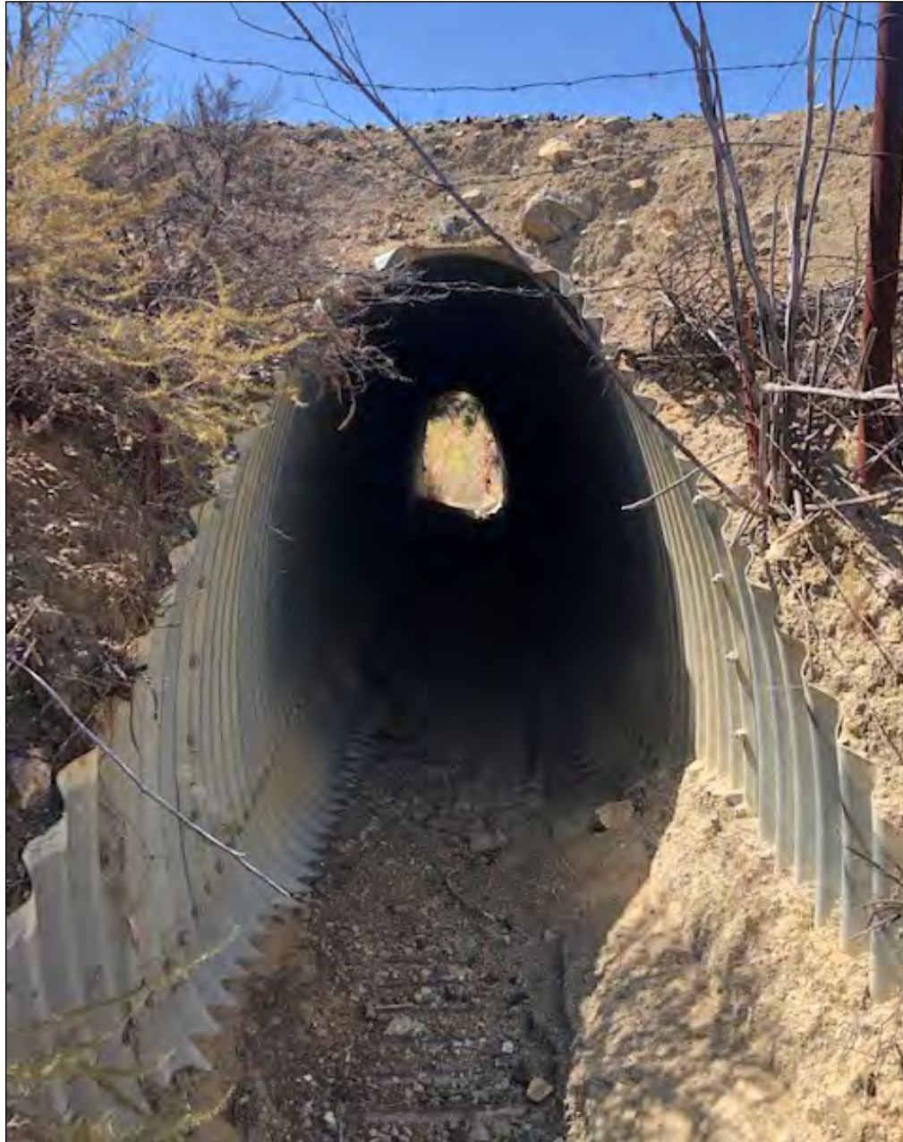
Figure 4-4 Culvert undercrossing, facing east.
