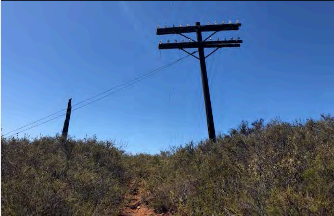
Figure 4-2 Power pole, facing west.
