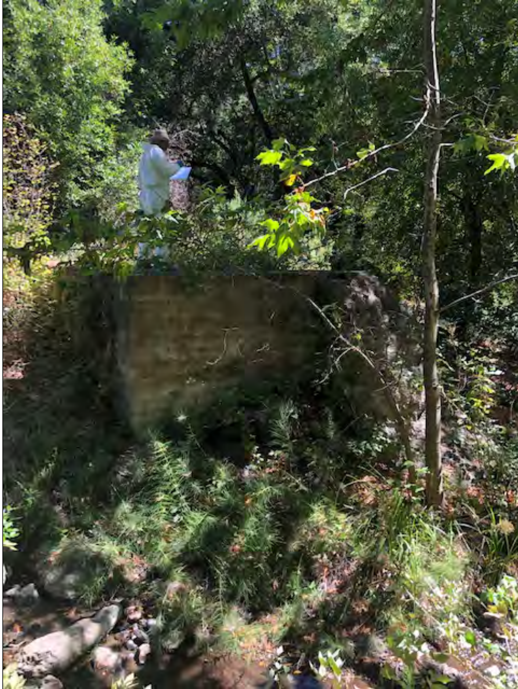
Figure 4-6 AE-4087-01H, Western segment of dam, facing east.
