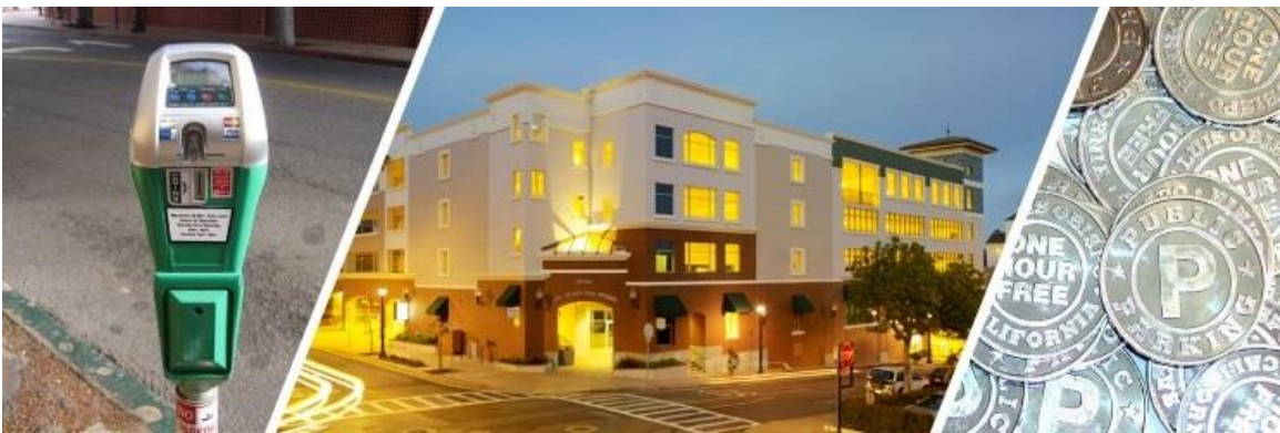
Morro Street & Palm Street Parking Structure
