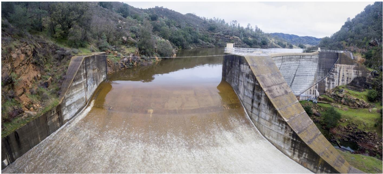
Salinas Reservoir Spillway.
