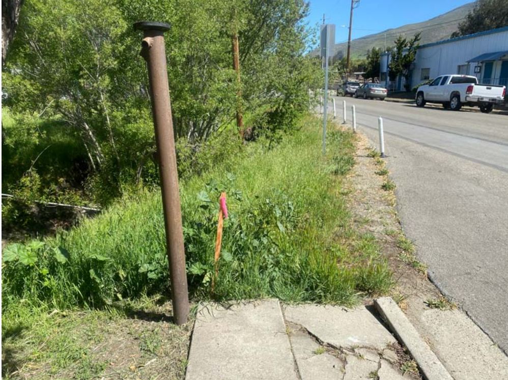
Photo 5. View from the southeast corner of the parcel looking north. Mc Millan Avenue is on the right. The road is actively eroding in this location.
