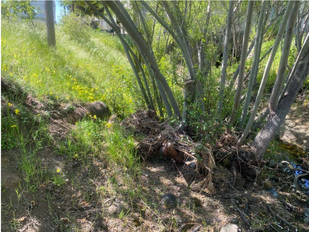
Photo 13. An outfall pipe into the channel is seen on the left. View is downstream. Note the racking of vegetation on the willow clump.
