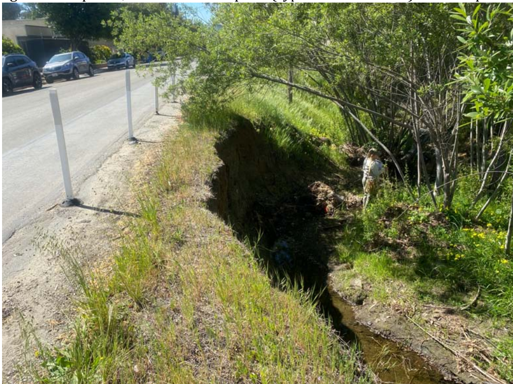
Photo 12. View of the eastern eroded bank along McMillan Avenue. A terrace within the channel is seen on the right.
