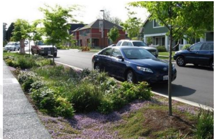
Green Infrastructure: Bioswale
