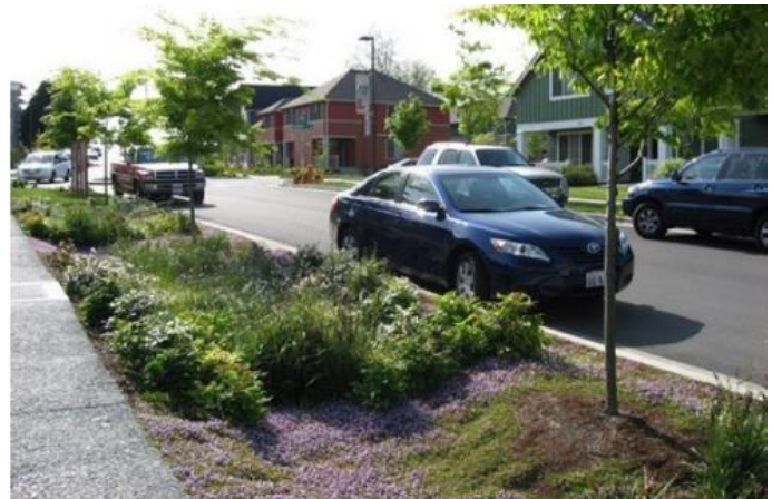
Green Infrastructure: Bioswale
