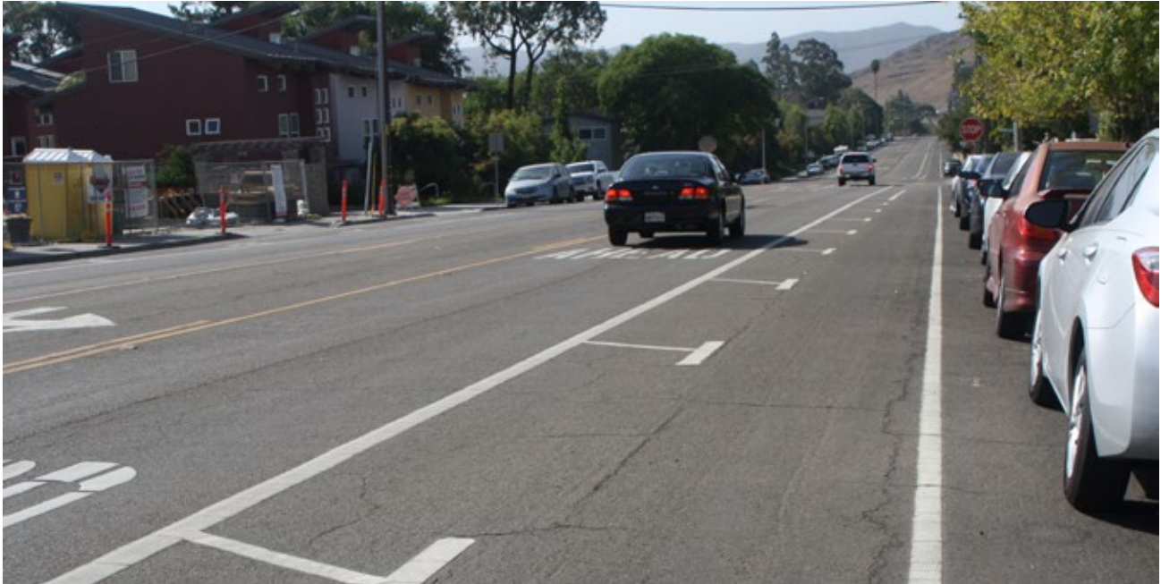
Buffered bike lanes transition into conflict markings. The use of additional pavement markings delineates space between vehicles and cyclists.
