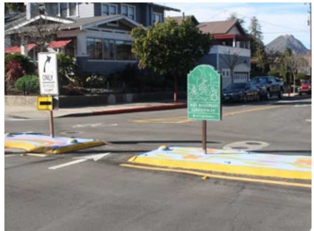
Chockers, planters, and curb extensions can also be used to restrict access to streets providing for slow-speed use instead of cut-through vehicle traffic.
