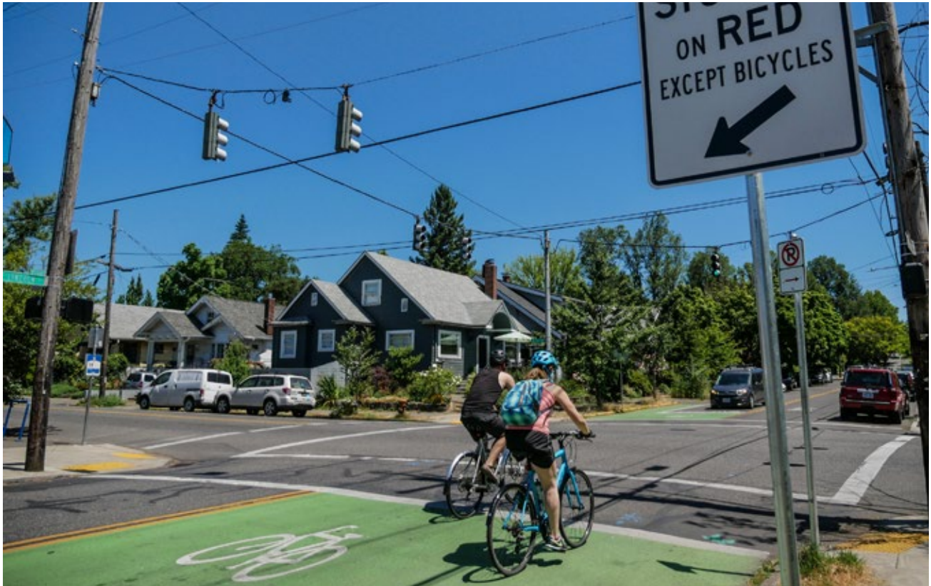
A bike box allows for cyclists to wait in front of queuing traffic, providing high visibility and a head start over motor vehicle traffic.
