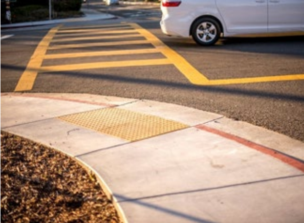
Diagonal curb ramps only recommended when right-of-way does not allow directional ramps.
