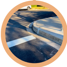
Curb Ramps Project Completed December 2021
