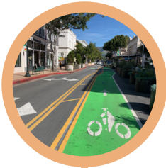
2022-23 Roadway Sealing Construction Ongoing
