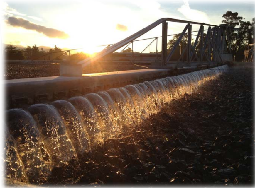
Water Resource Recovery Facility
