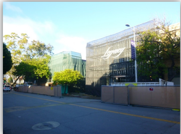
Chinatown Commercial Development under Construction
