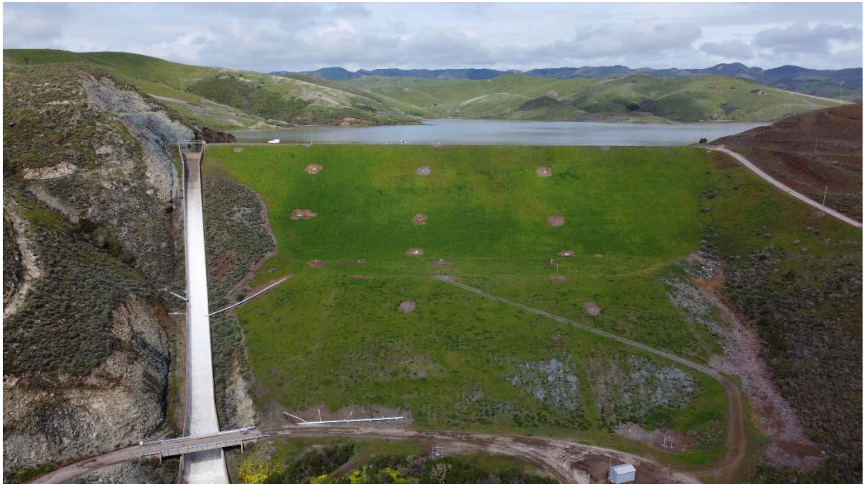
Whale Rock Reservoir and Spillway.
