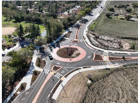
New Roundabout at Orcutt Rd & Tank Farm Rd
