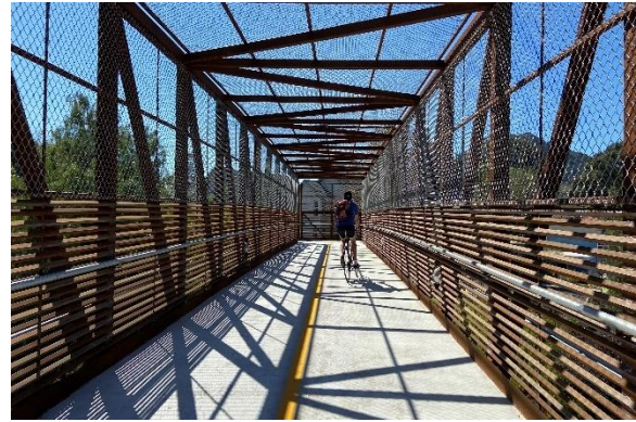
Railroad Safety Trail from Taft Street to Pepper Street
