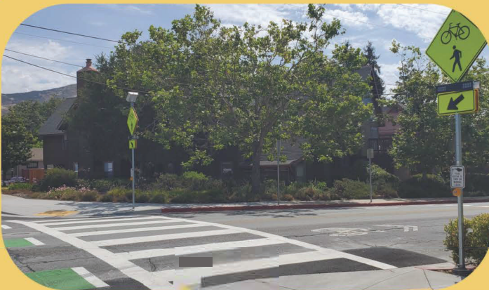
Pedestrian crossing improvements at Johnson, South, Broad, Madonna, Foothill, and Osos Streets
