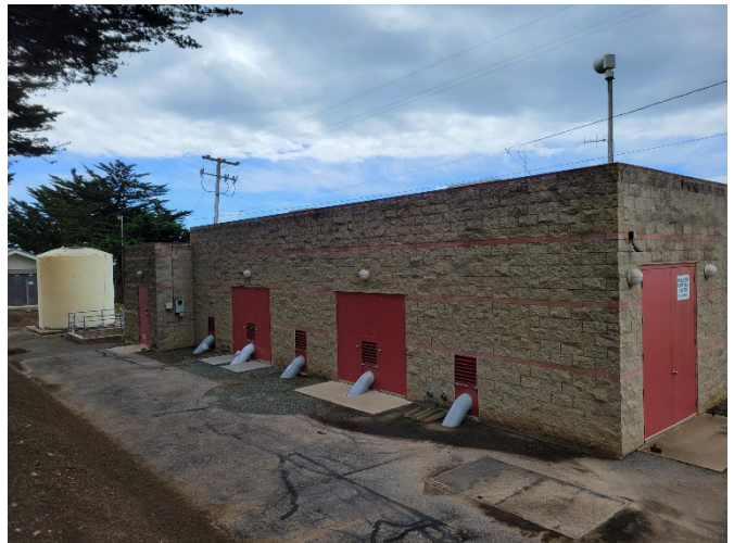
Pump Station A
