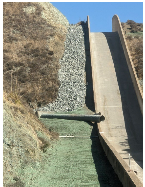
Completed Spillway Underdrain Repairs
