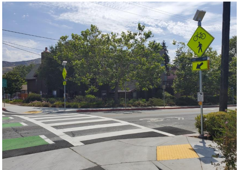
New Pedestrian Crossing Improvements
