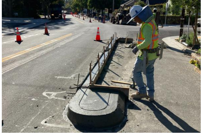
North Chorro Neighborhood Greenway Construction
