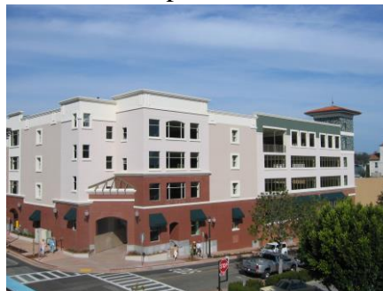
919 Palm St. Parking Structure
