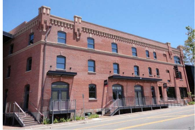
Channel Commercial Company, 1880 Santa Barbara Avenue, 1912. Photo 2013; source City of San Luis Obispo.
