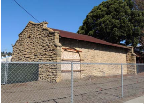
Old Gas Works, 280 Pismo Street, 1902. Photo 2013; source Historic Resources Group.
