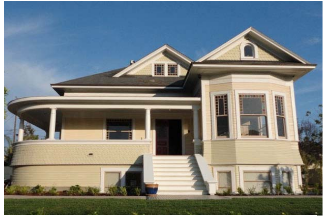
Sandercock House, 535 Islay Street, 1910. Photo 2013; source City of San Luis Obispo.
