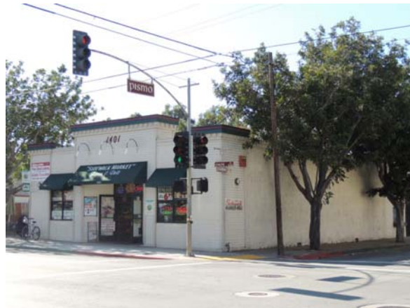
1401 Osos Street. Source: Historic Resources Group.
