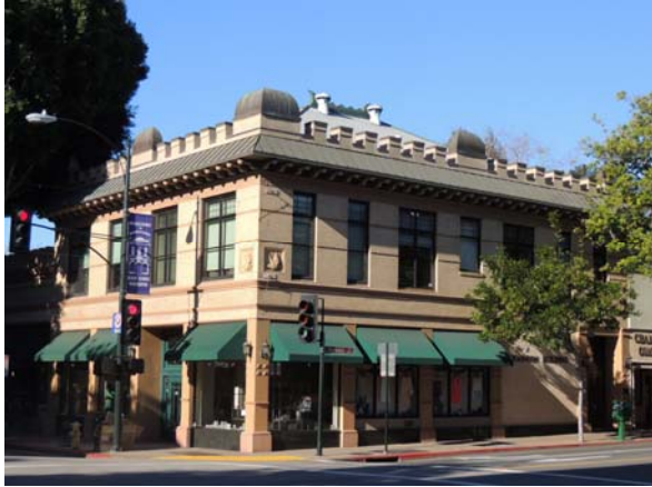
Johnson Building, 796 Higuera Street, 1903-1904. Photo 2013; source Historic Resources Group.
