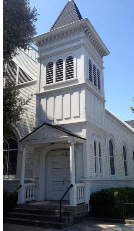
First Baptist Church, 1301 Osos Street, 1907. Source: City of San Luis Obispo.
