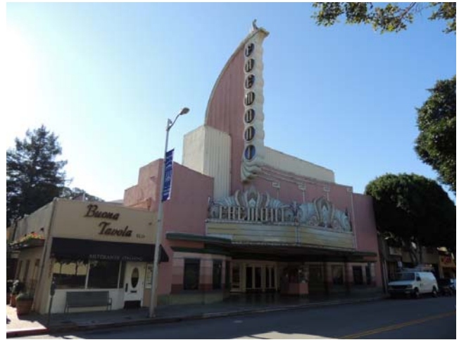
Fremont Theatre, 1941. 1035 Monterey Street. Source: Historic Resources Group.
