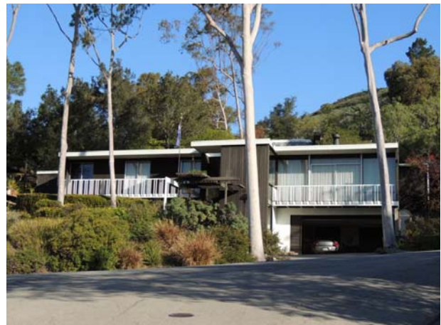
Ken Schwartz House, 201 Buena Vista Avenue, 1964. Photo 2013; source Historic Resources Group.
