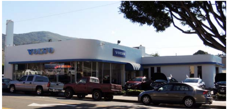
1219 Monterey Street. Source: Historic Resources Group.
