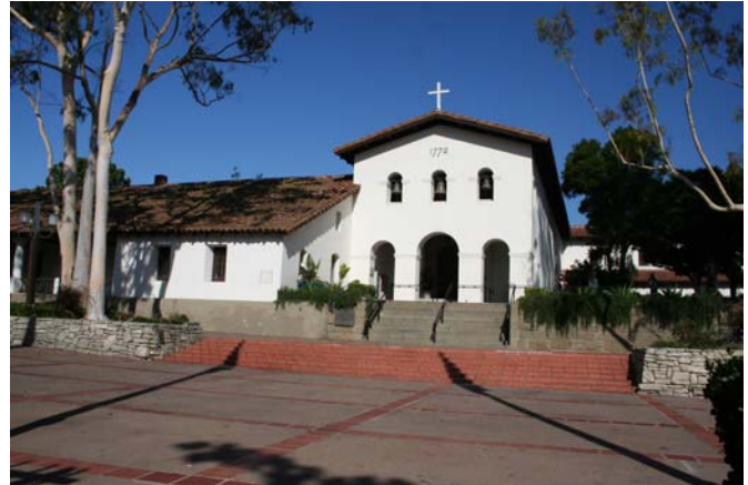
Detail of Mission Plaza in 2012. Source: Historic Resources Group.
