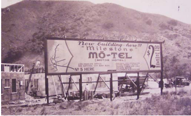
Milestone Mo-tel under construction, 2223 Monterey Street, 1924. Source: Huntington Library, San Marino.
