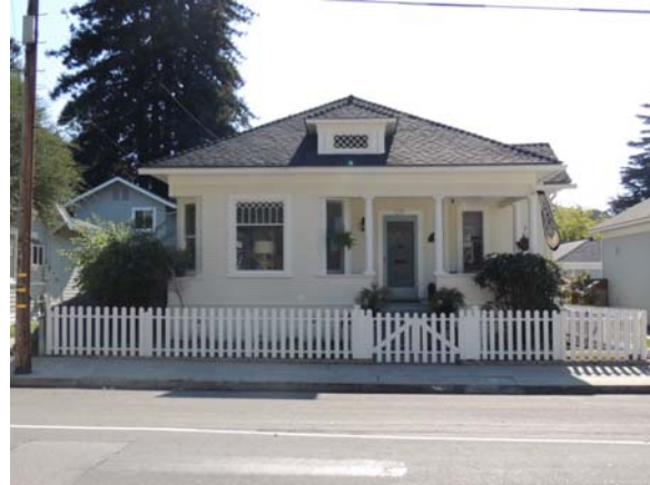
1211 Pismo Street, 1908. Source: Historic Resources Group.
