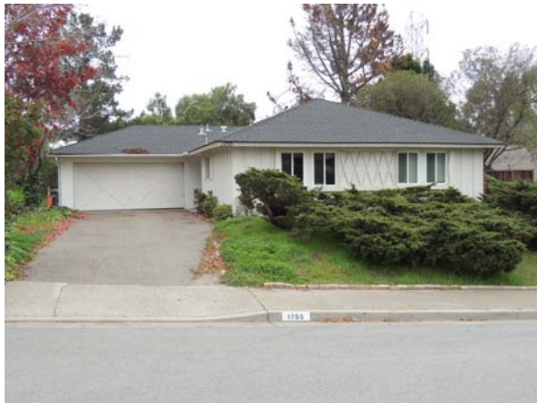
1755 Tanglewood. Source: Historic Resources Group.
