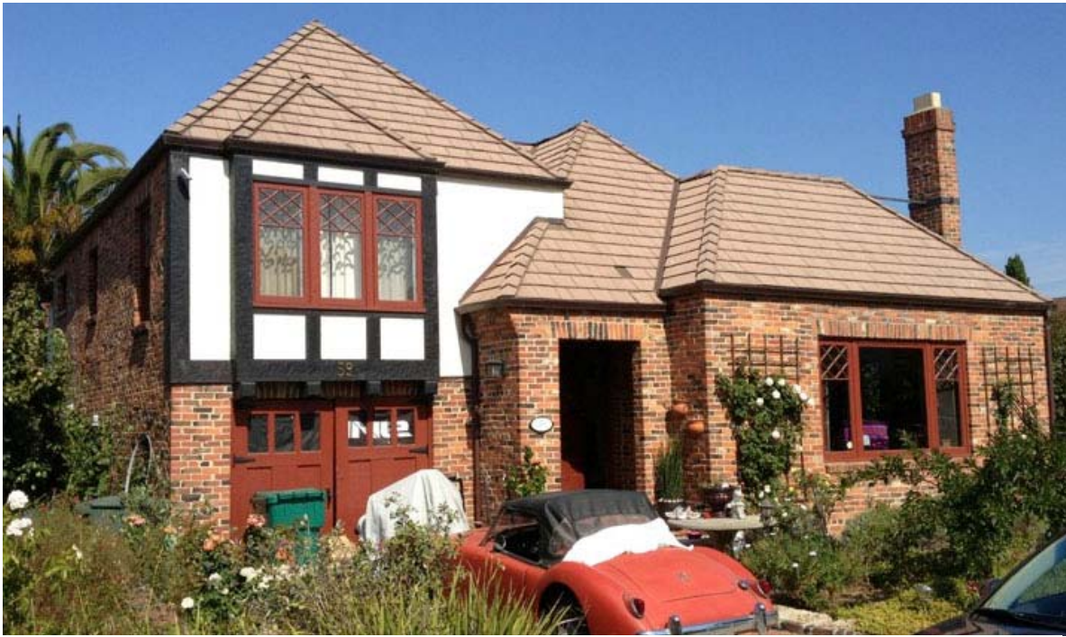
Dunne House, 59 Benton Way, 1927. Photo 2013; source City of San Luis Obispo.
