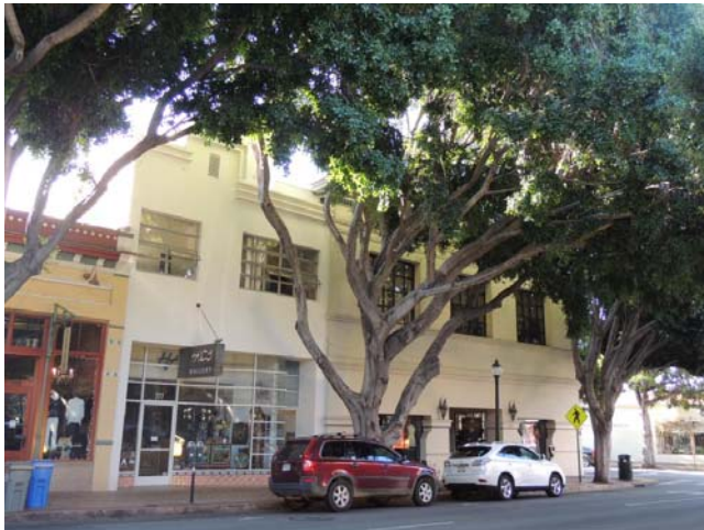
Doton Building, 1931. 777 Higuera Street. Source: Historic Resources Group.
