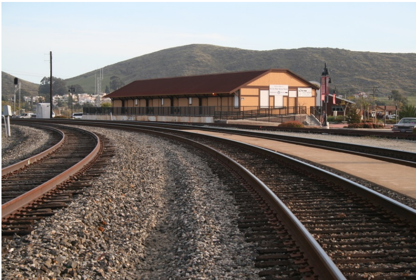
Southern Pacific Railroad Warehouse, 1940 Santa Barbara Avenue, c. 1895. Photo 2013; source Historic Resources Group.
