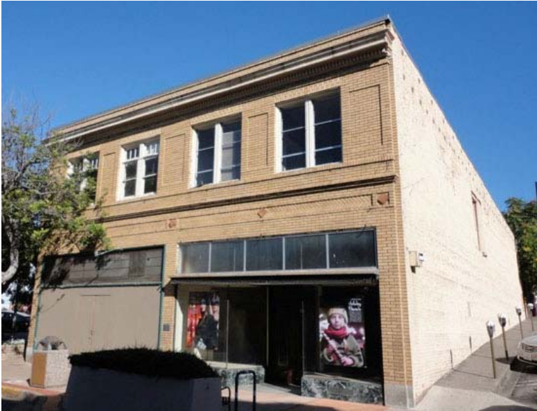
Muzio's Grocery, 868 Monterey Street, 1912. Muzio's moved from its original location to a new storefront in the Wineman Hotel on Higuera Street in 2010; it has since closed. Photo 2013; source City of San Luis Obispo.
