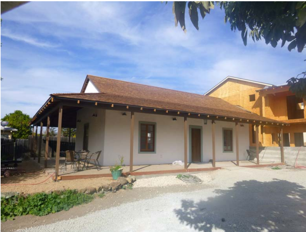
Mancilla/Freitas Adobe, 868 Chorro Street, c. 1800-1850. Photo 2014; source City of San Luis Obispo.
