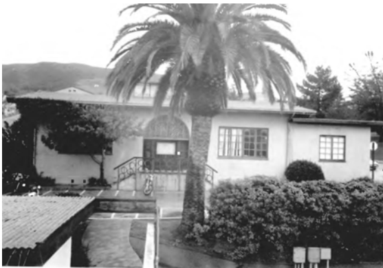
Powerhouse, Cal Poly San Luis Obispo, NE corner of S. Perimeter and Cuesta Avenue, 1909. Photo 1993; source National Register nomination form.
