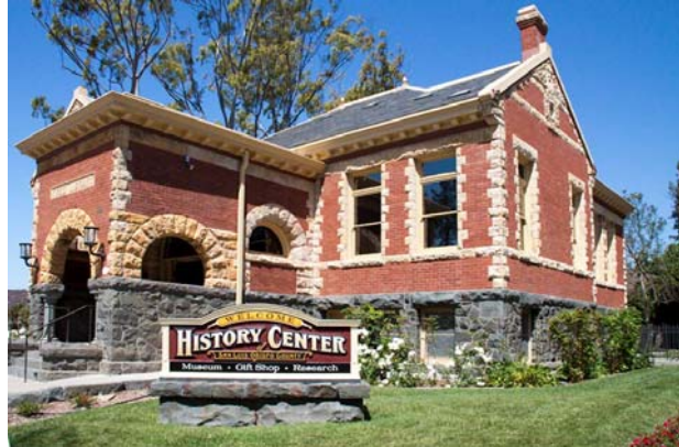
Carnegie Library, 696 Monterey Street, 1905. Photo 2013; source Historic Resources Group.
