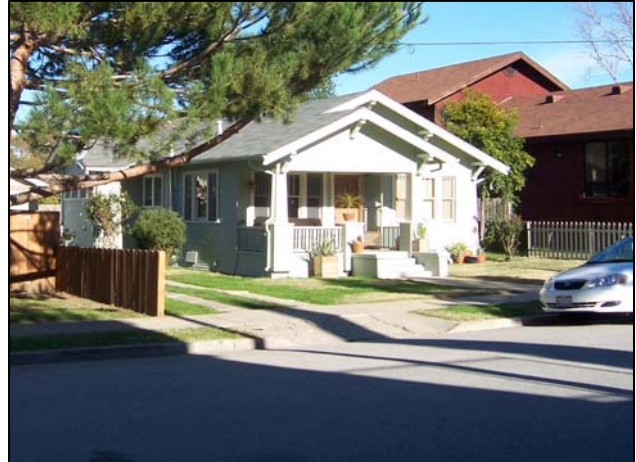
1034 Church St, South Elevation
