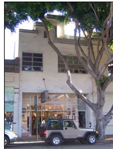
Doton Building, 777 Higuera Street, North Elevation
