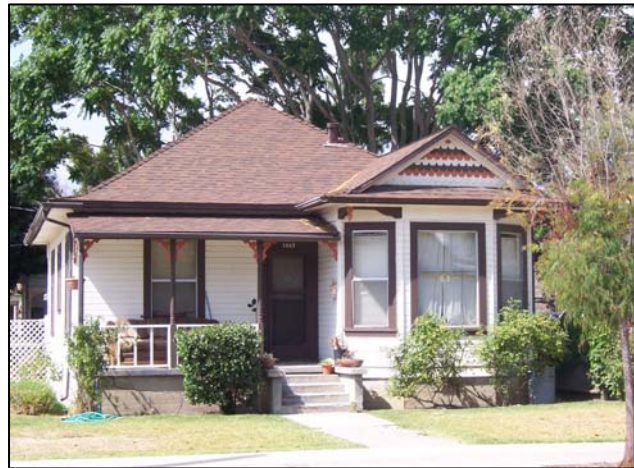
1543 Morro Street, East Elevation
