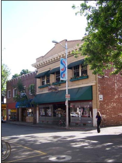
Smith Building and Union Hardware Building, 1119 and 1129 Garden Street, East Elevation
