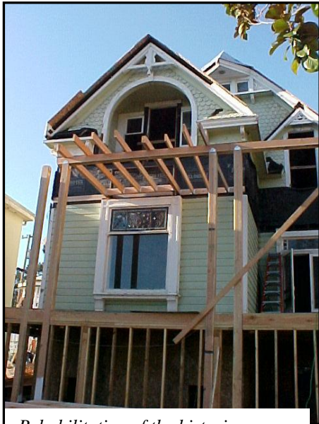
Rehabilitation of the historic Righetti House, 2007
