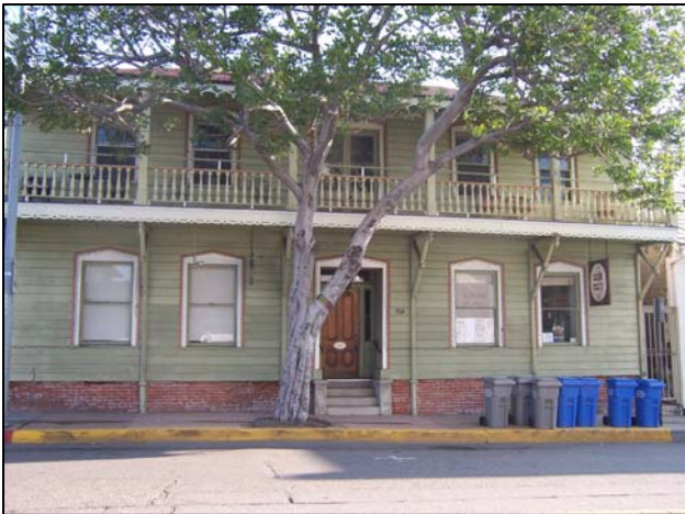
Sauer/Adams Adobe, 964 Chorro Street, West Elevation
