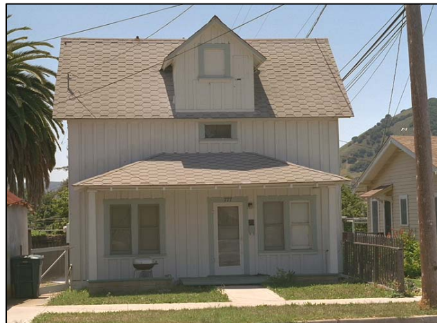
777 Johnson Avenue, East Elevation
