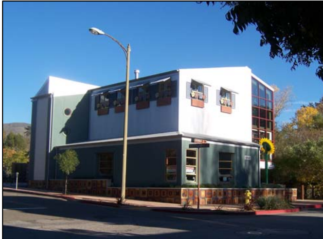
1010 Nipomo Street, South and West Elevations
