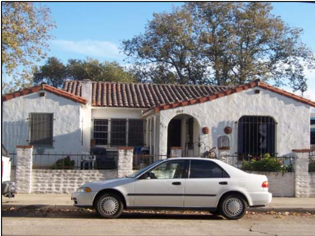
469 Dana Street, North Elevation
