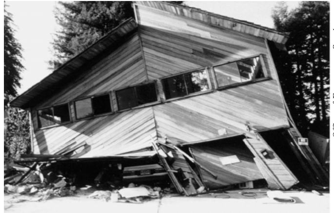
Figure 29 - This mountain home was built over a garage, and its walls were not strong enough to withstand an earthquake.
