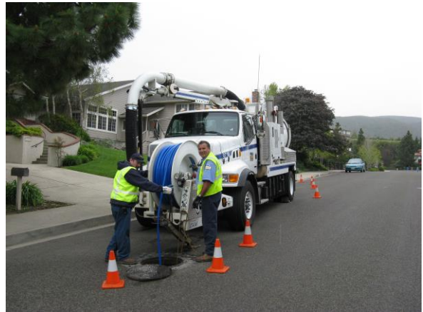
City Wastewater Collection staff cleaning a sewer main using the Vac-con.
