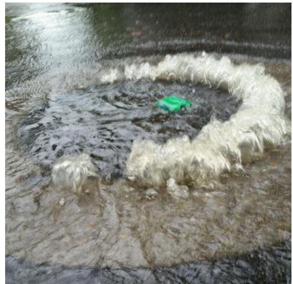
Sanitary sewer overflow at manhole, 2018.
