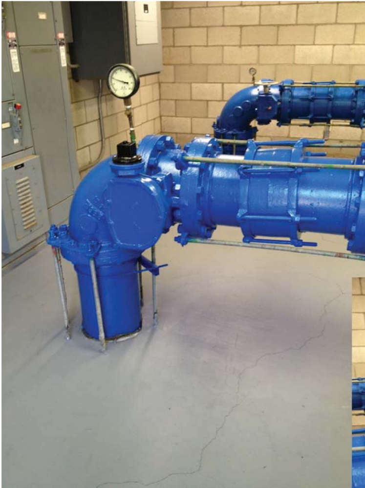
Ferrini Pump Station - Interior
