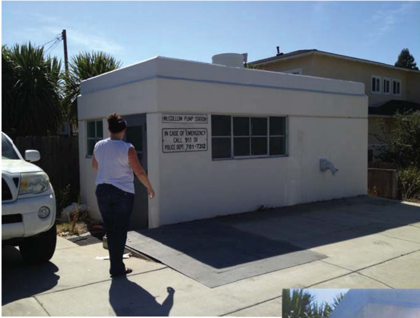
McCollum Pump Station - Exterior
