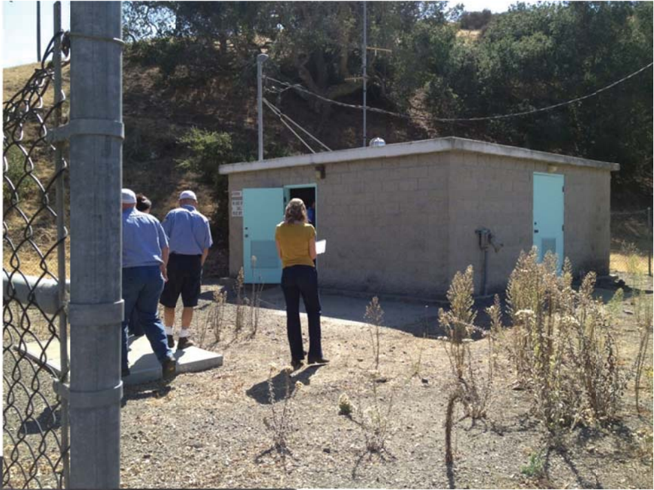
Ferrini Pump Station - Exterior and Interior
