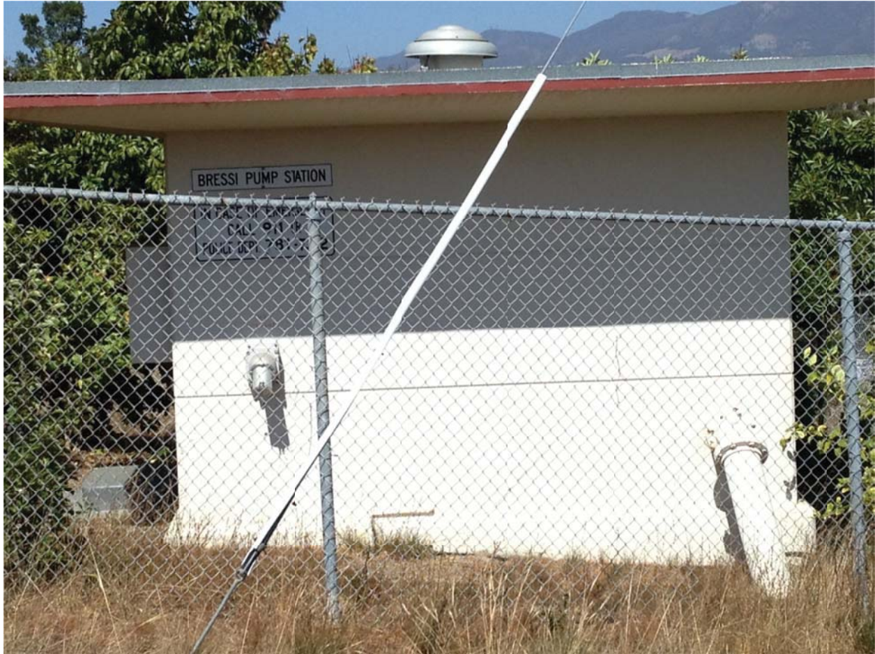
Bressi Pump Station - Exterior
