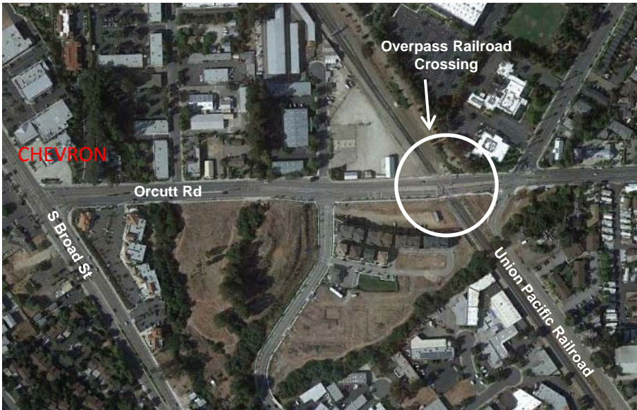
12-1. Existing Overpass Railroad Crossing
