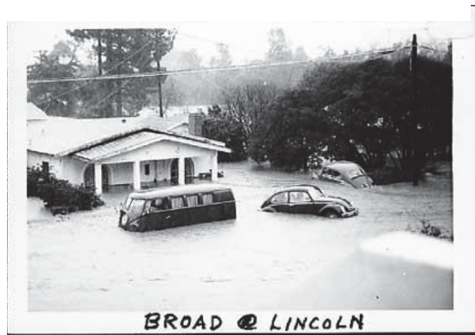
Figure 4-13 1973 Flooding at Broad and Lincoln in the City of San Luis Obispo
